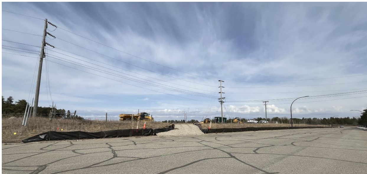
Work has begun at the Beltrami County Jail site on Pioneer Street SE., April 9, 2025.
