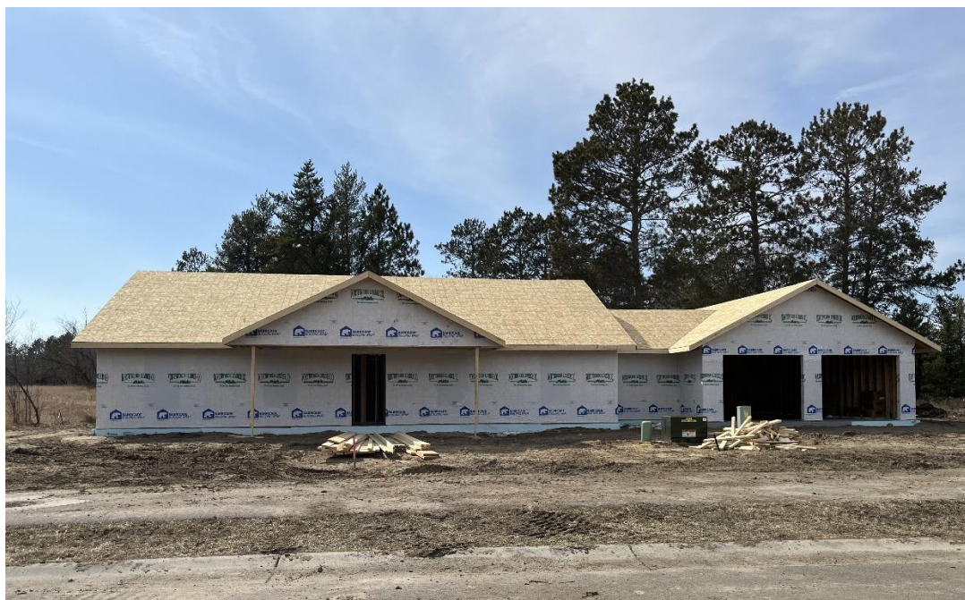
New home construction, Beartooth Ave SW, April 9, 2025.
