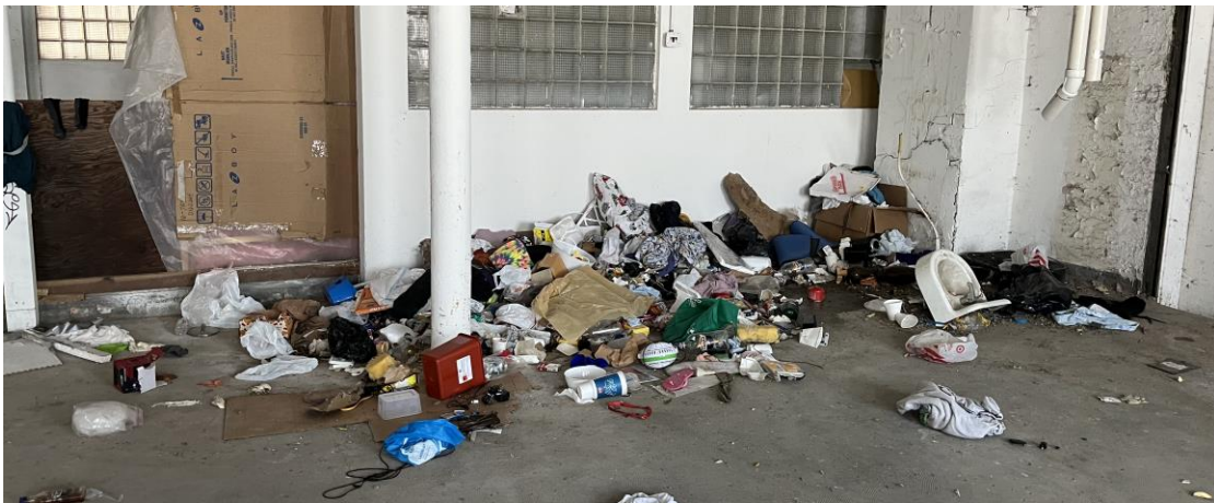
Trash pile on main floor.
