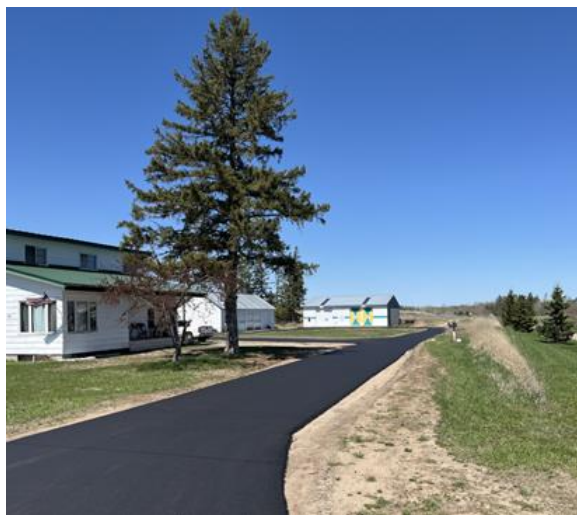
Project on Anne St NW that recently completed paving.
