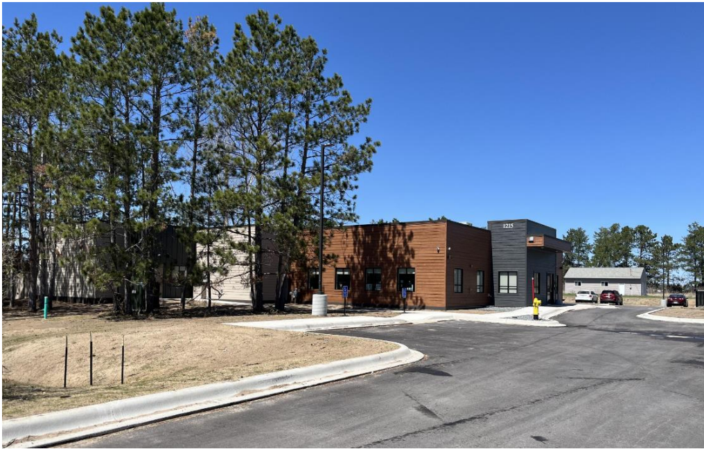
The Northwoods Battered Women's Shelter is near completion.
