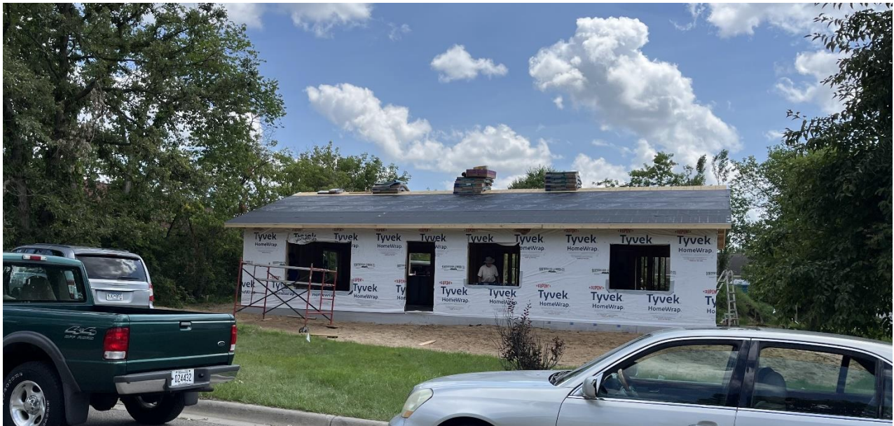
Habitat for Humanity house construction, 19th St NW – July 9, 2025
