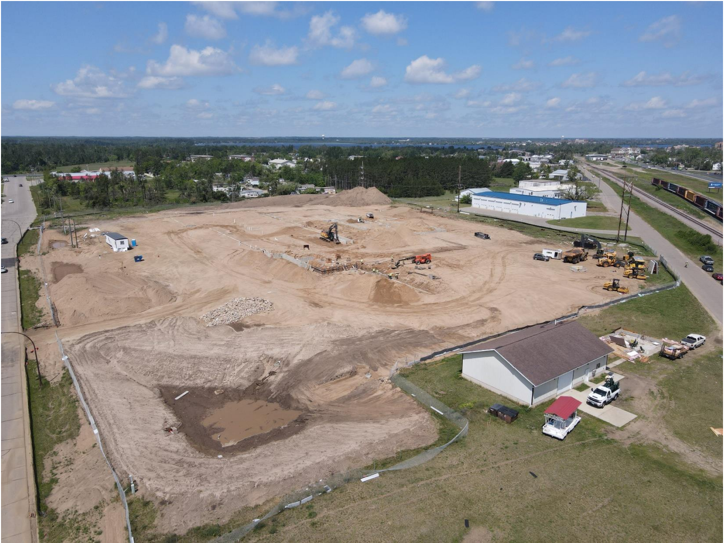
Beltrami County Adult Corrections Center construction site, June 23, 2025
