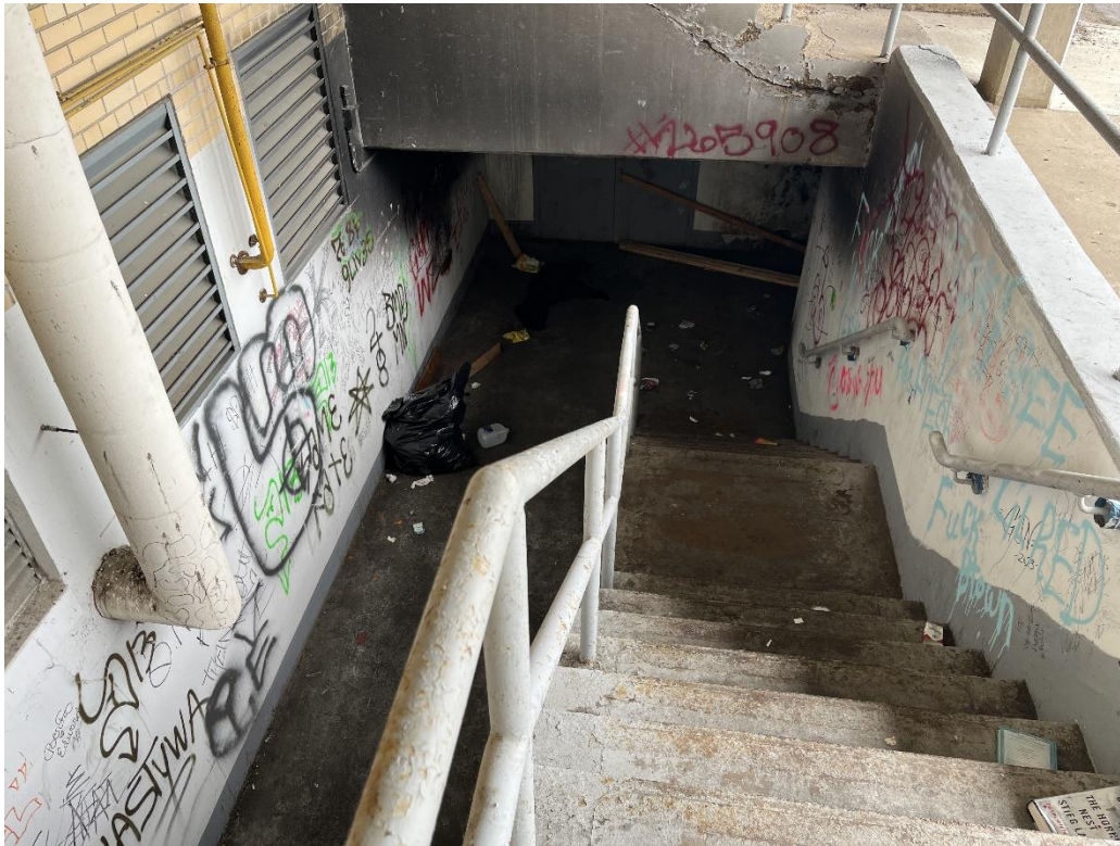
Basement access, old Federal Building.
