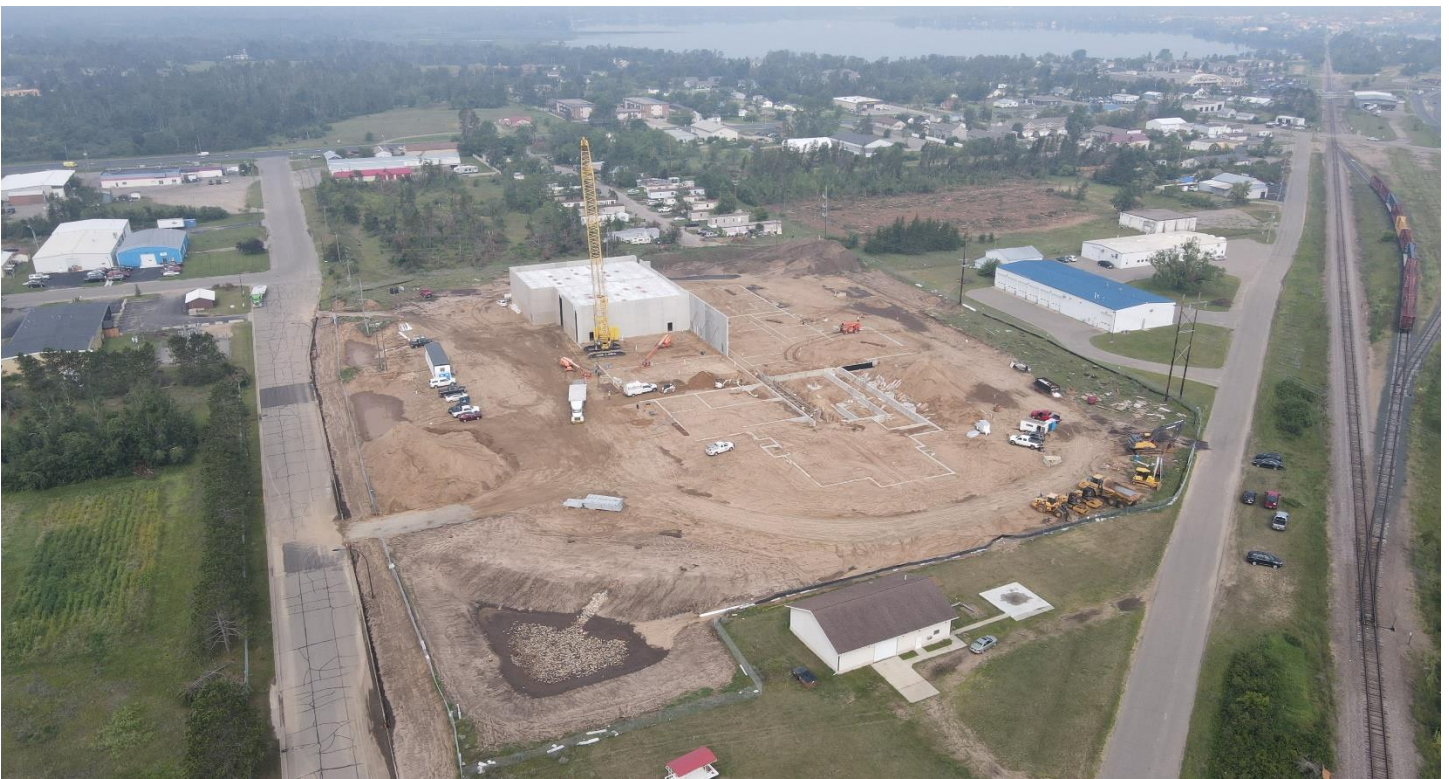
Beltrami County Adult Corrections Center construction site, July 24, 2025
