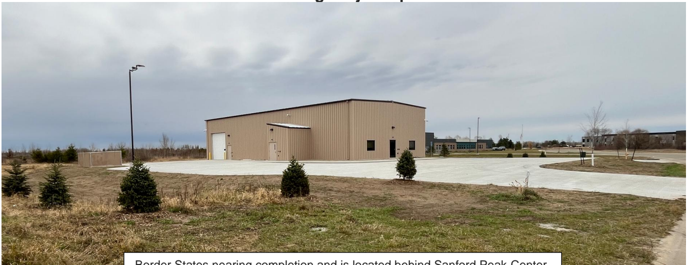
Border States nearing completion and is located behind Sanford Peak Center.
