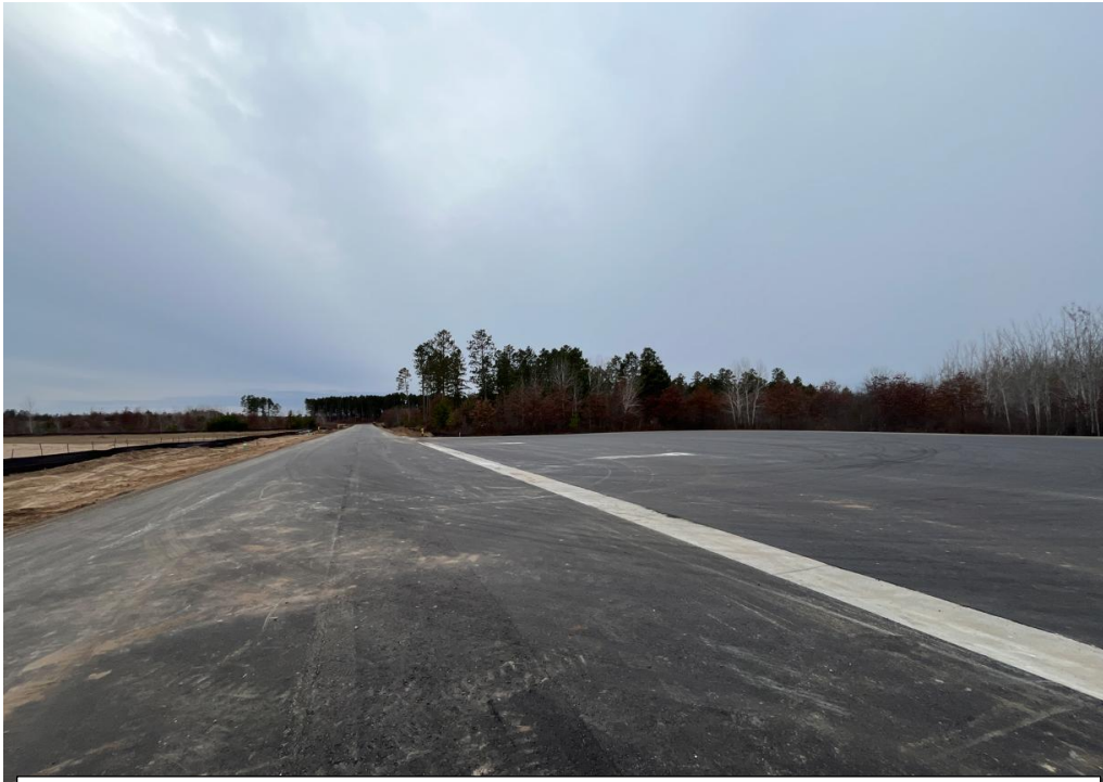
Airport planning area 3's phase I infrastructure completion (Looking west).
