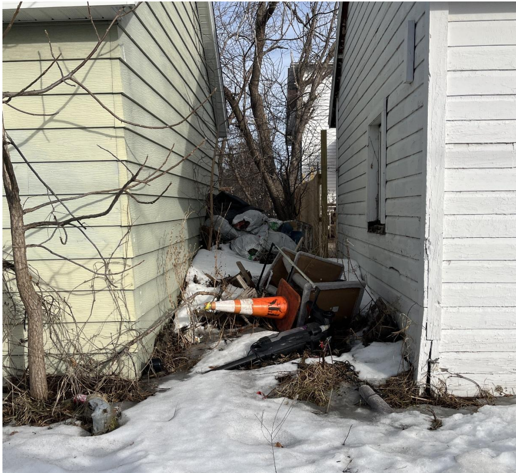
Bagged household trash and furnishings creating a Section 28-402 violation, March 4, 2026.
