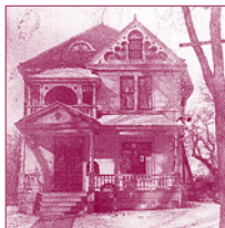
Above: the porch at Elmwood after restoration; right, a historic view.
