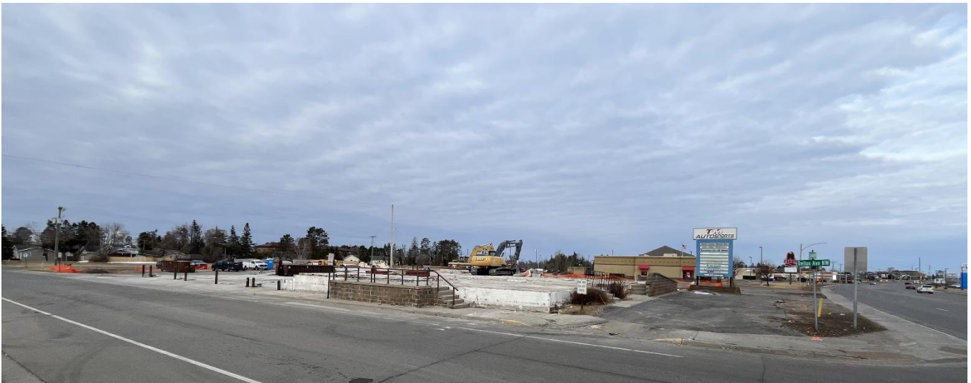
Demolition at the future Les Schwab Tire Center site, April 1, 2026
