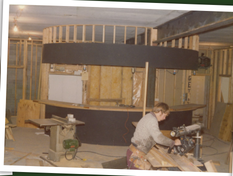
Construction of the main bar fall of '74
