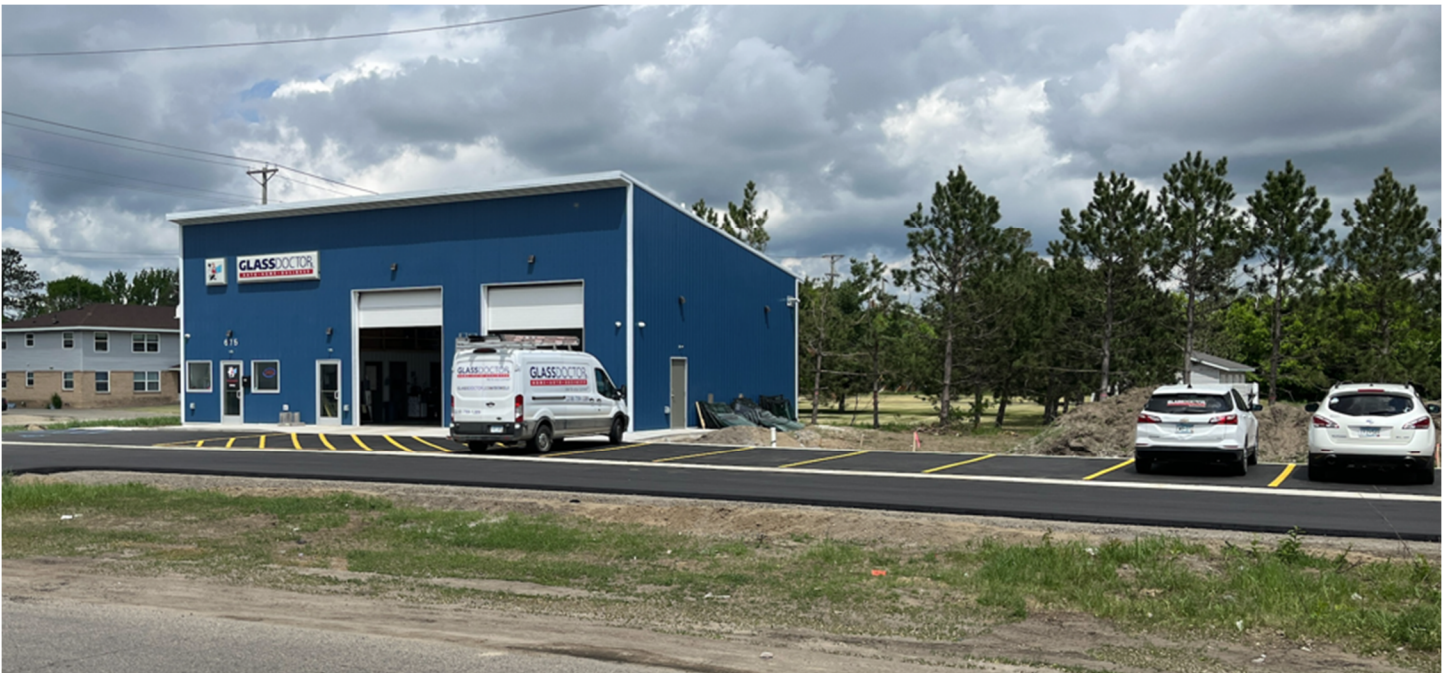
Parking Lot completed Glass Doctor site, June 4, 2026
