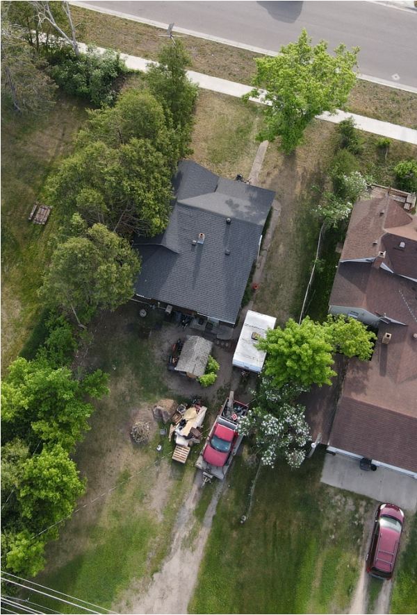
Photo showing exterior storage violations - June 2, 2026
