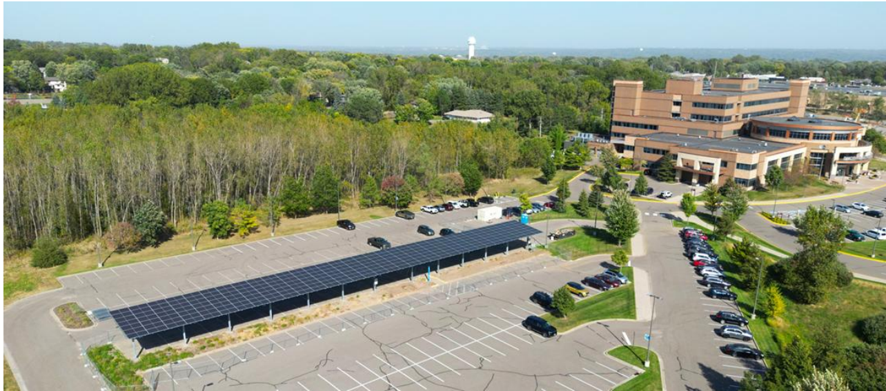
Northern Service Center South St. Paul
