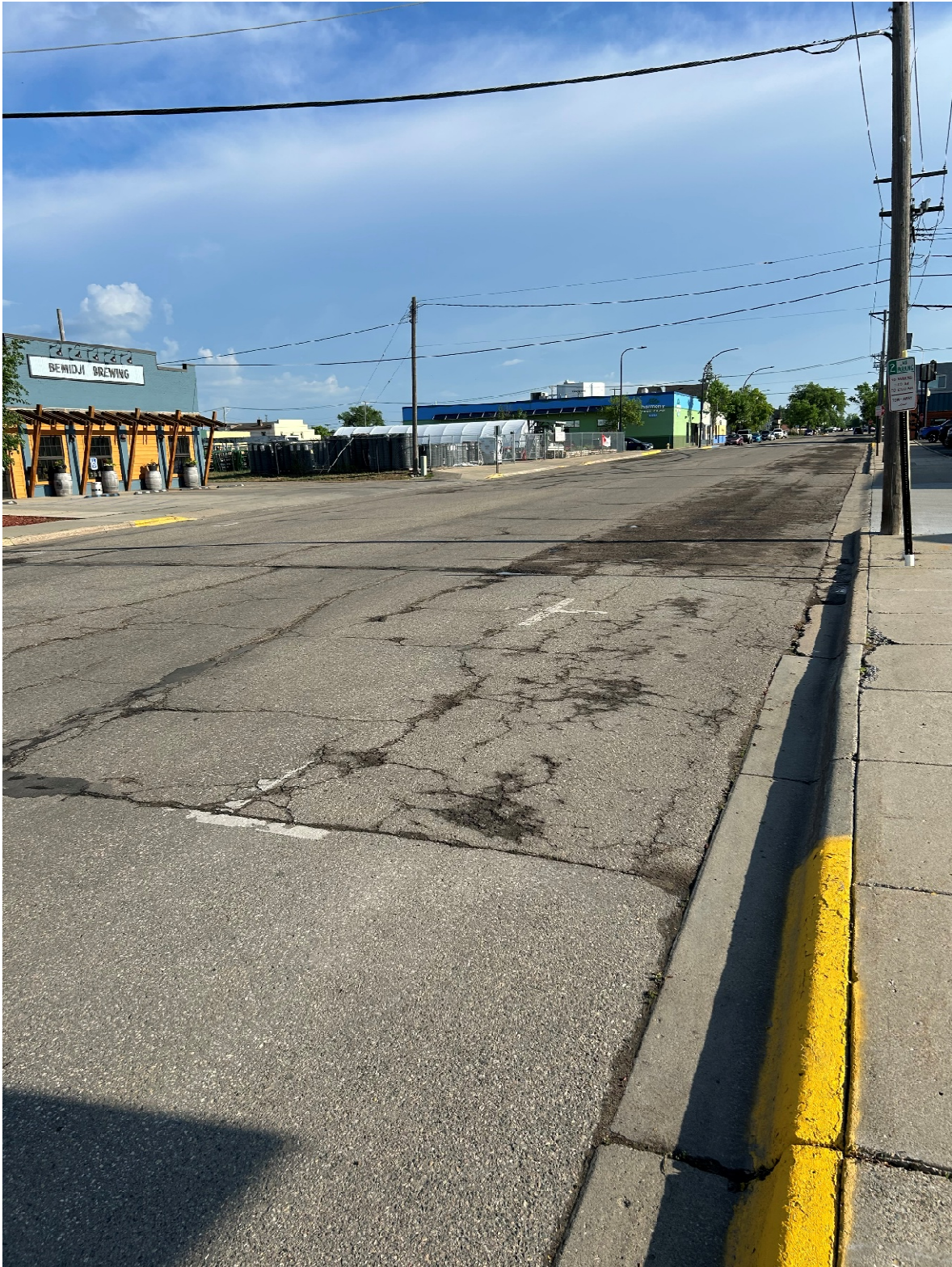
Existing conditions – on America Avenue NW looking north toward 3 rd Street NW
