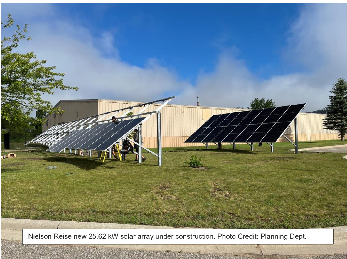
The newly installed 39.28 kW solar array for the warming house next to the rink. Photo Credit: Planning Dept.
