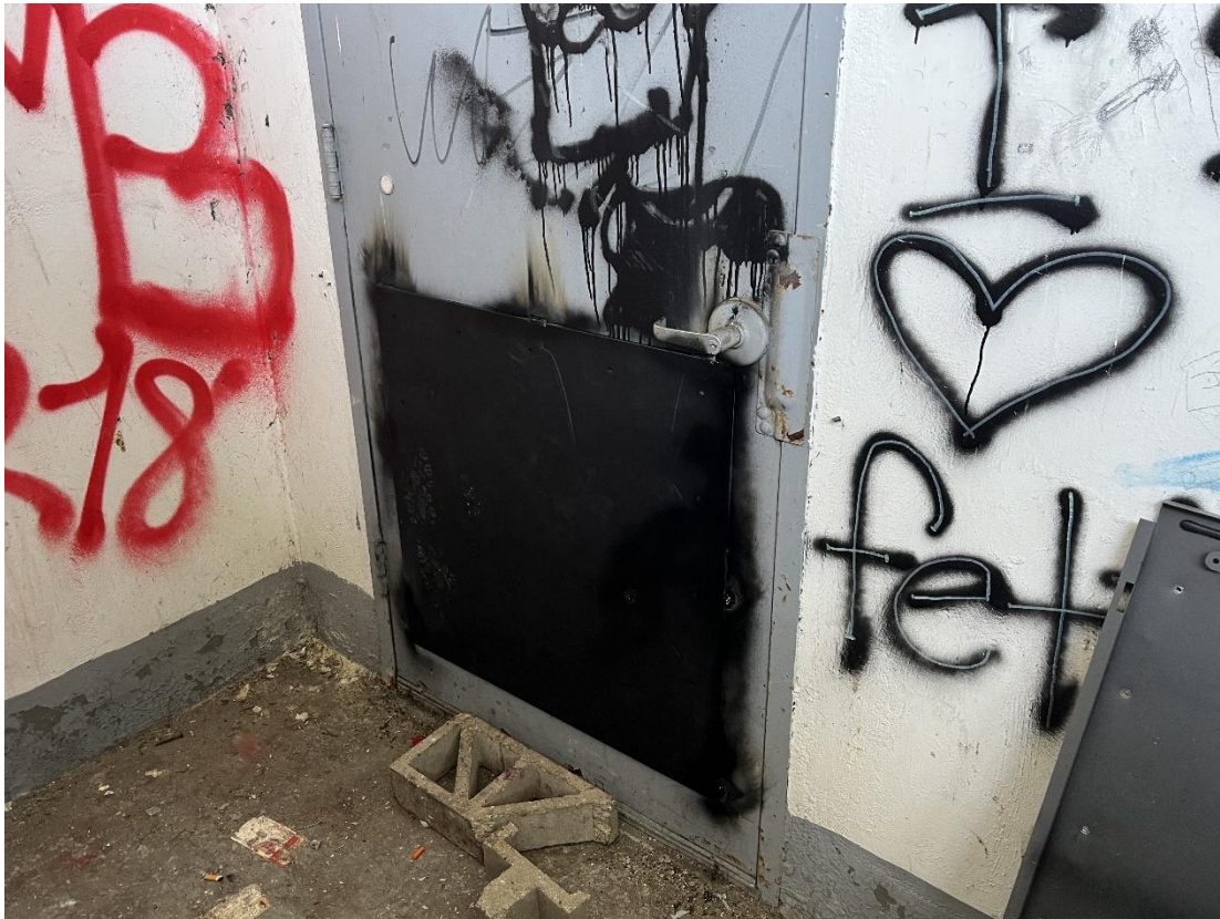
Basement door access to the Federal Building patched , June 22, 2026
