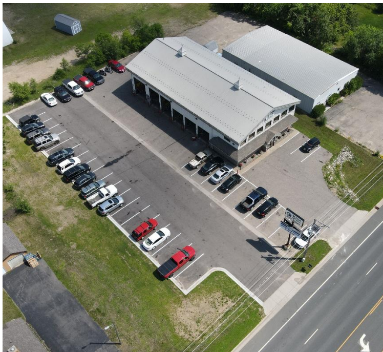
Completed Motor Works Parking Lot, July 9, 2026
