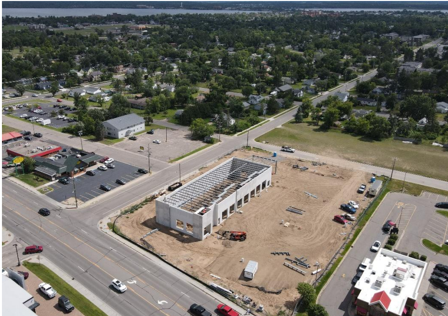
Les Schwab construction site, August 4, 2026
