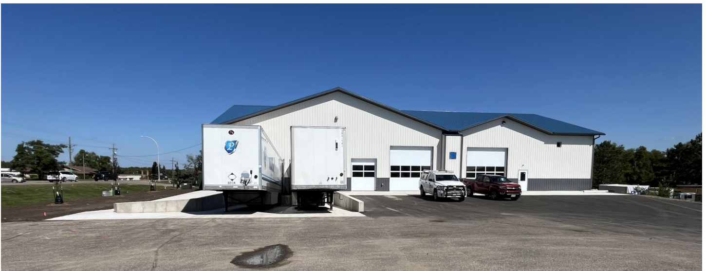
Peterson Sheet Metal Aug. 31, 2026. Construction appears complete. DA will be reviewed to verify completion of the project.
