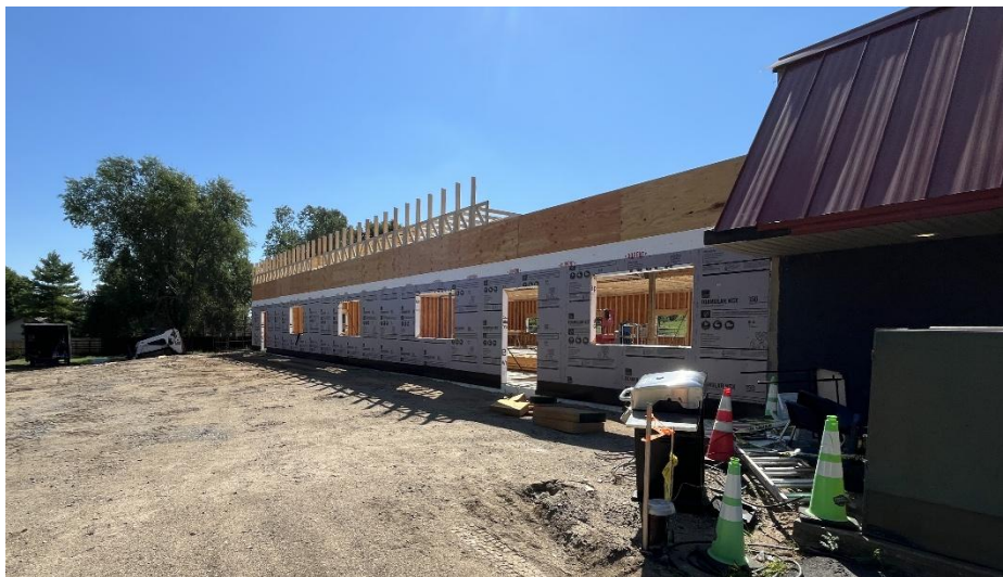
Voyageur Expeditionary High School construction site, August 31, 2026
